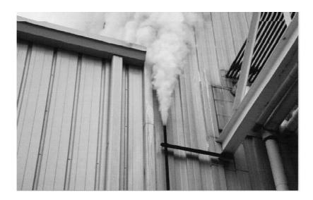
**Look at the flash vents along the high pressure distribution system.** That flash energy that is floating off into the atmosphere could be returned to the boiler plant instead.
